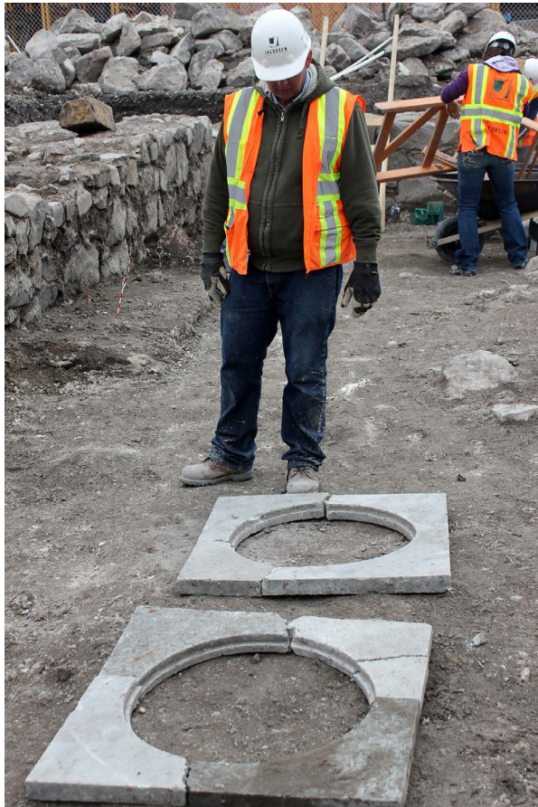
Figure 4.20. Rich Talbot, director of OPA, examines refit stone frame (left); it is likely that these framed the heating grates after steam heating was installed in the building (ca. 1900) (images courtesy of OPA).
