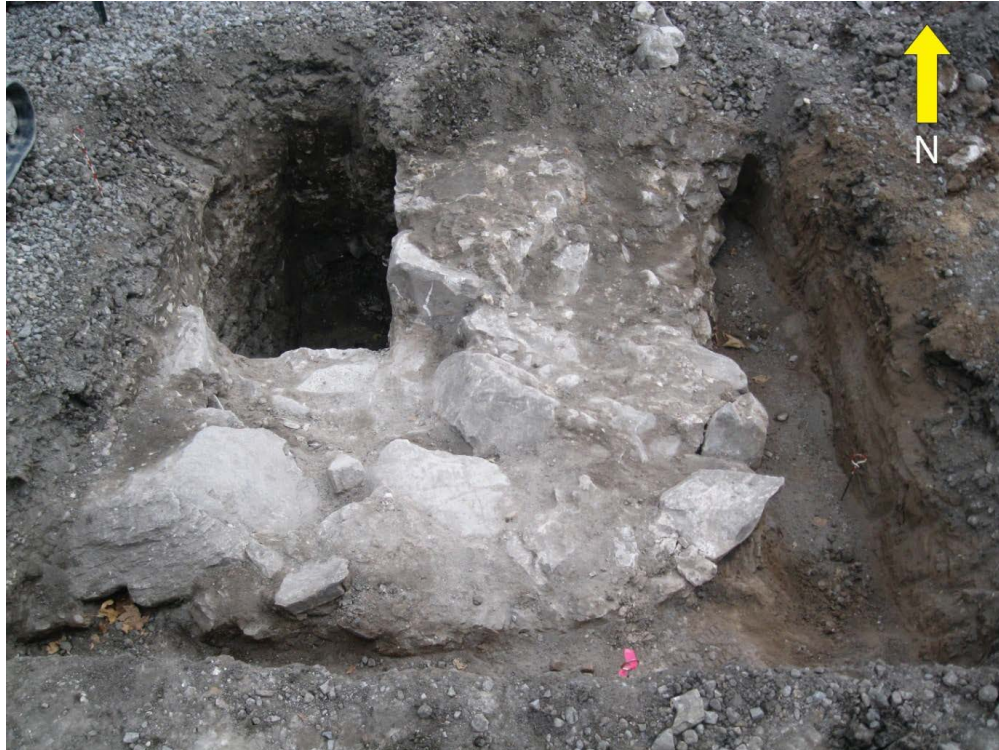
Figure 4.5. Photograph of initial test pit showing the southeast corner of the OPT foundation (image courtesy of OPA).
