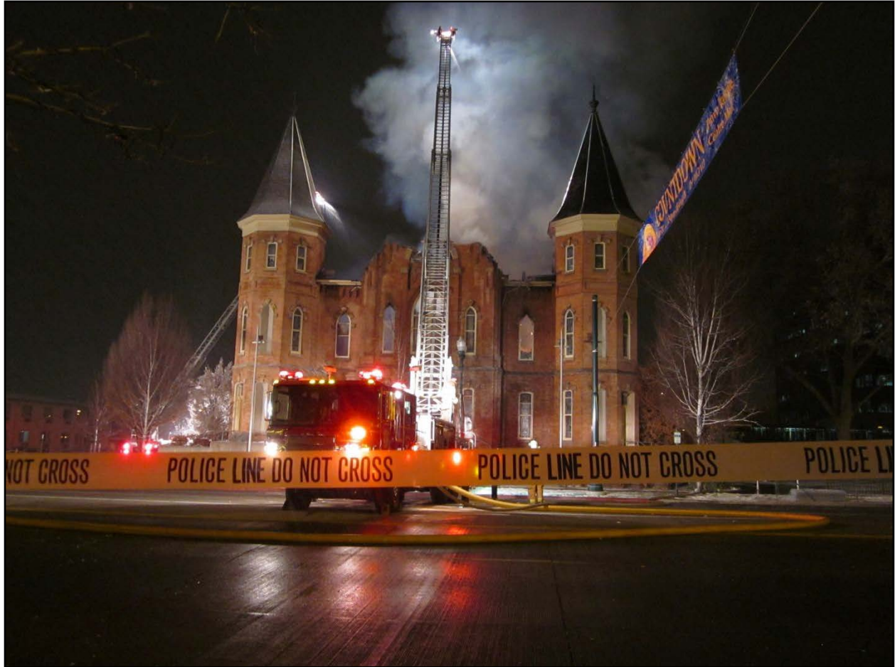
Figure 1.1. Fire crews working to put out the fire at the historic Provo Tabernacle, December 17, 2010 (photo courtesy of Provo resident Alison Broadbent).
